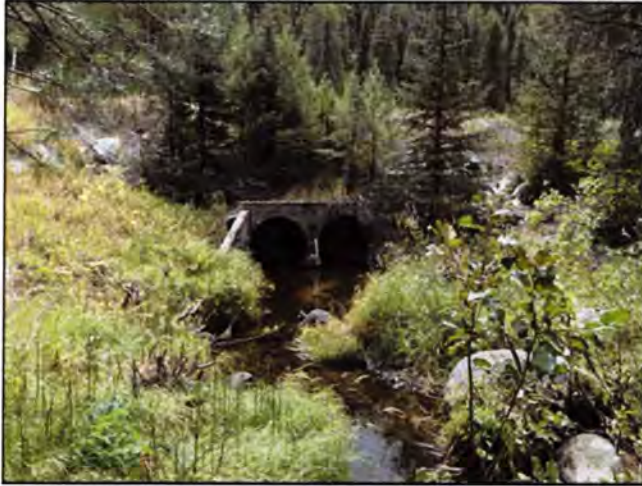
Bogus Creek Culverts
